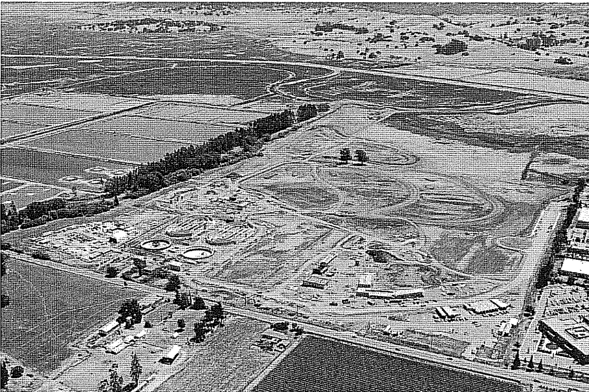
These are aerial photos of early construction on the City's Ellis Creek Water Recycling Facility, which will provide superior protection of public health and the environment. The top is from 2006 and the bottom is from 2007.
