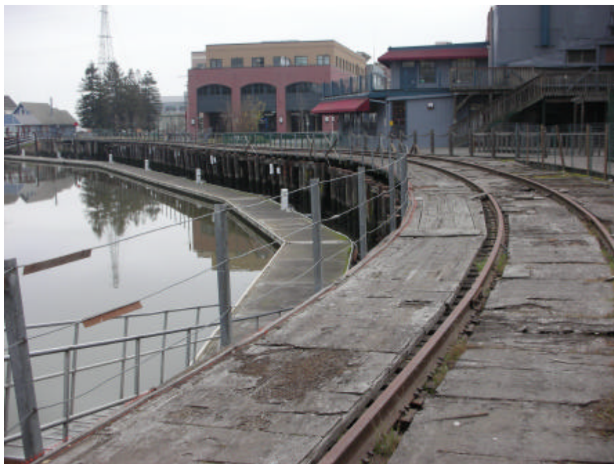
Figure 3: Trestle Overview, Looking East
