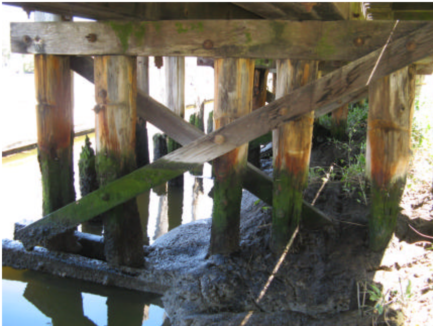
Figure 4: Typical Bent (Bent 29, looking east)
