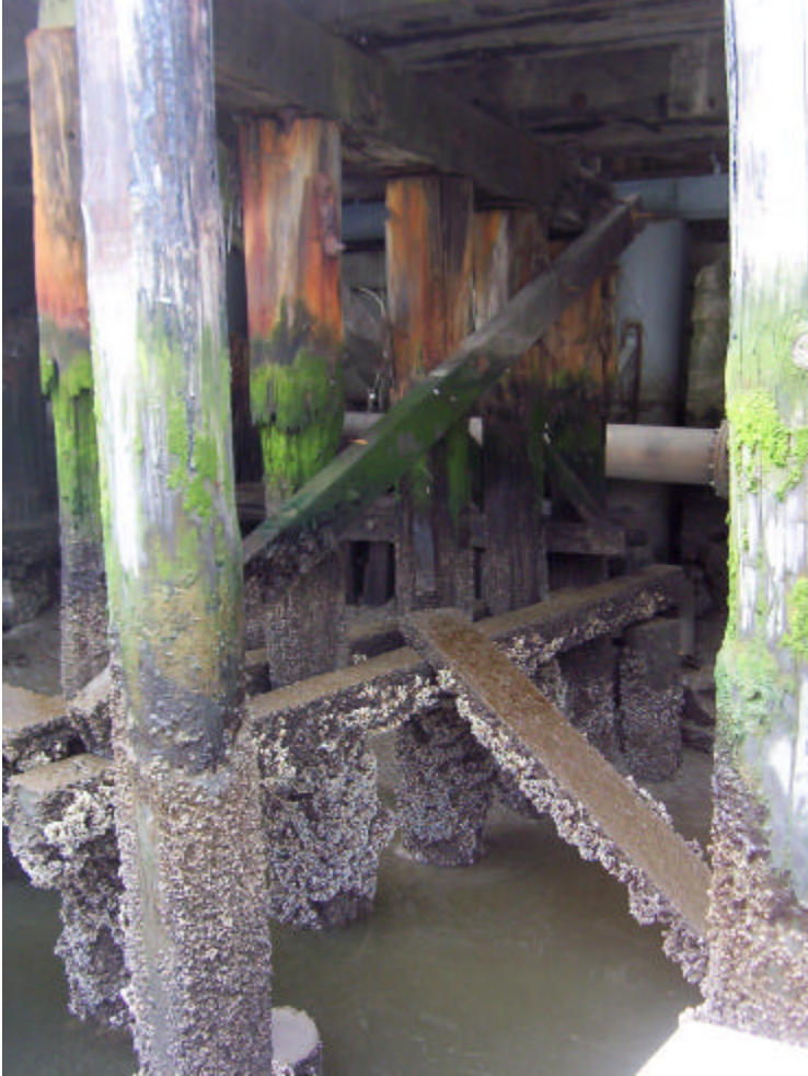
Figure 6: Typical Marine Growth (Bent 16)
