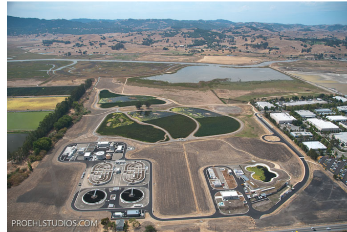
Aerial of Ellis Creek Water Recycling Facility
