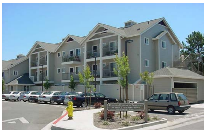
Lieb Senior Apartments – 22 units
